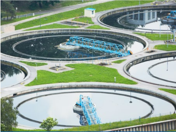
Utilize ultra-sonic sensing technology for level in water reclamation basins.
