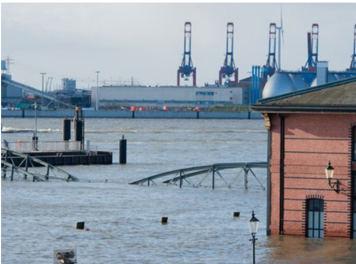
Monitor water level during and after flood events.
