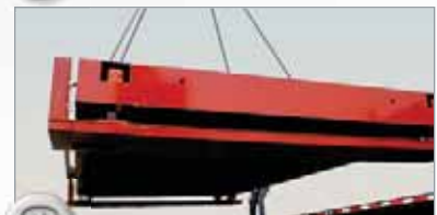
2 Unload and set modules.
