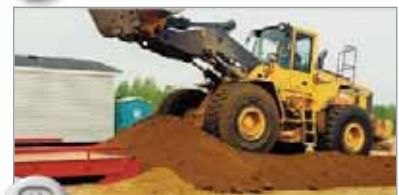
3 Backfill to bulkheads and finish ramps.
